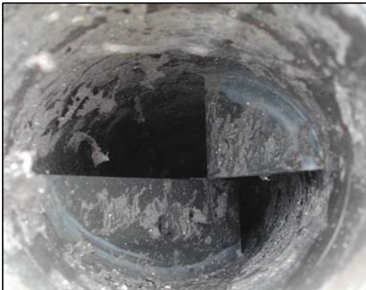
Statiflo Sludge Blender after 90 hours
